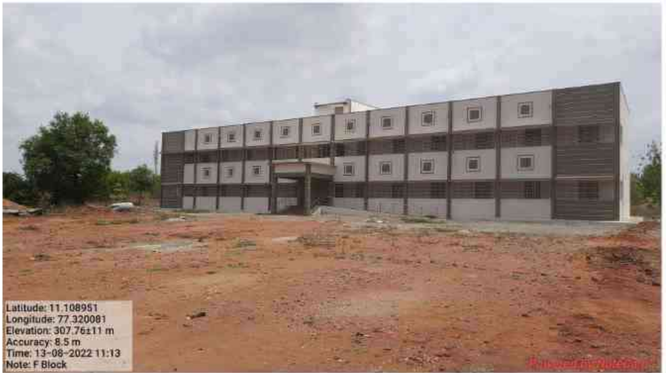
NEWLY CONSTRUCTING F BLOCK
